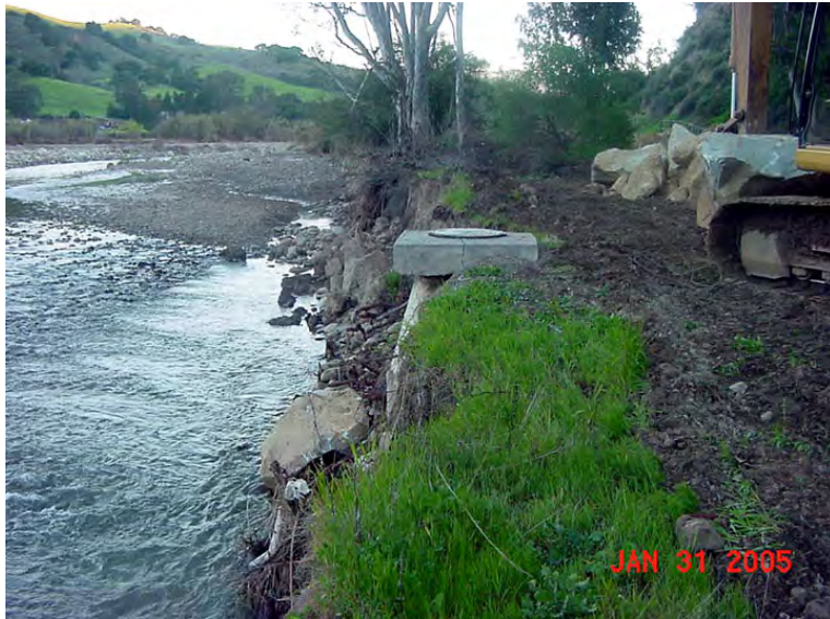
Sewer Manhole on the Ventura Riverbank During 2005 Flood
