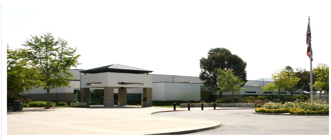
The Todd Road Jail, a pre- and post-sentencing facility near Santa Paula
