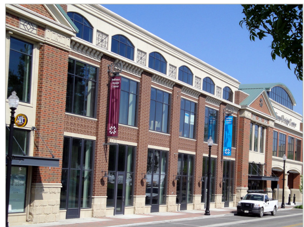
Example of a commercial building that breaks a long façade into multiple vertical segments.
