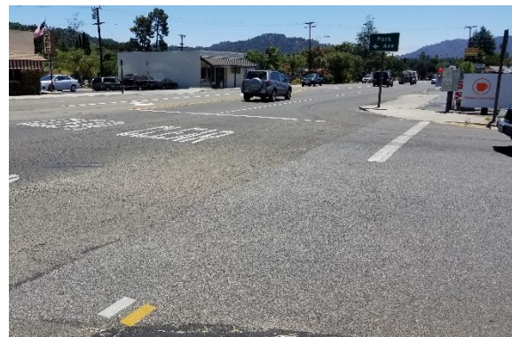
Figure 19: Incomplete limit lines and missing pedestrian crosswalk
