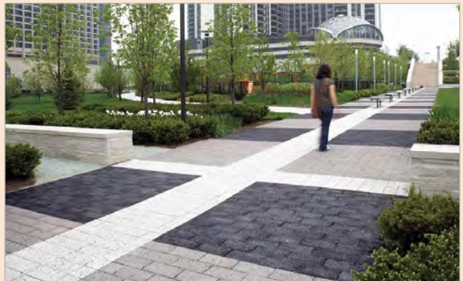
A simple, formal paving pattern made by using different paving materials. This example embodies the intent of the guideline.
