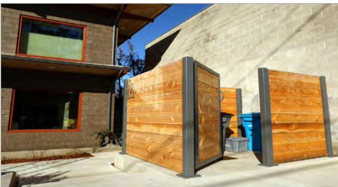
Image 6.19. A screened trash enclosure.
