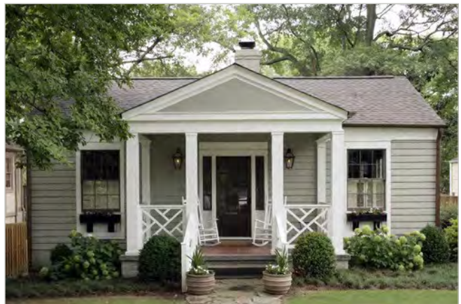
Image 6.8. A porch addition that uses materials and design matching to the existing home.
