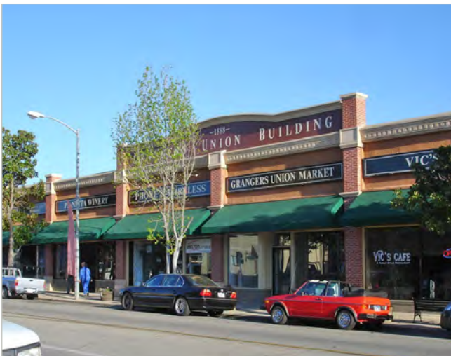
Image 6.13. A "Main Street" commercial building with a flat roof screened by parapet walls.
