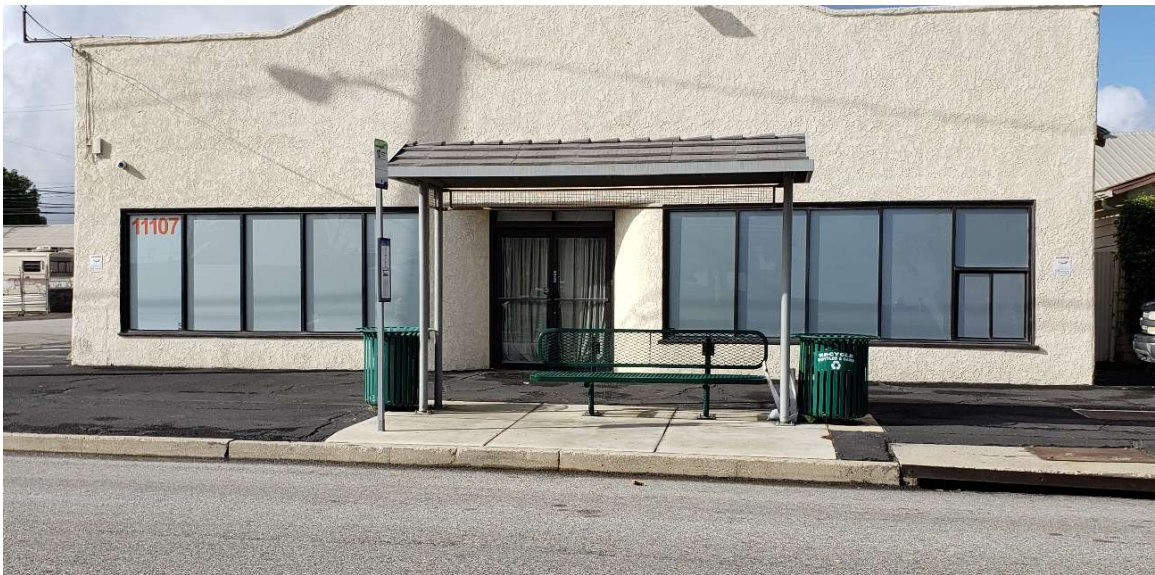
Benches, shelters, and trash receptacles at this bus stop on Violeta Street, near Los Angeles Avenue, help create a more comfortable transit experience.
