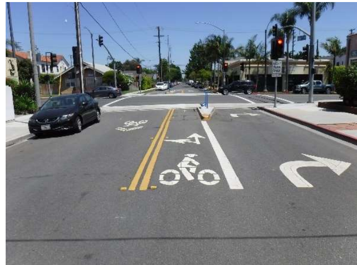
Bicycle Boulevards incorporate traffic calming measures such as diverters to maintain low vehicular volumes.
