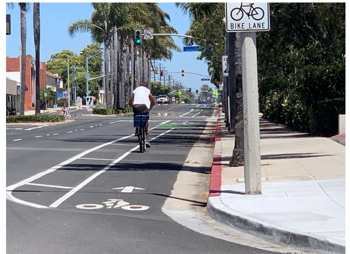
Class II bike lanes provide dedicated space on the roadway for people riding.
