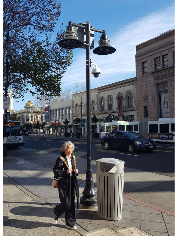
In addition to standalone pedestrian-scale lighting, street lights can be fitted to include pedestrian-scale fixtures that illuminate the walking area, while higher, vehicle-scale street lights illuminate the roadway.
