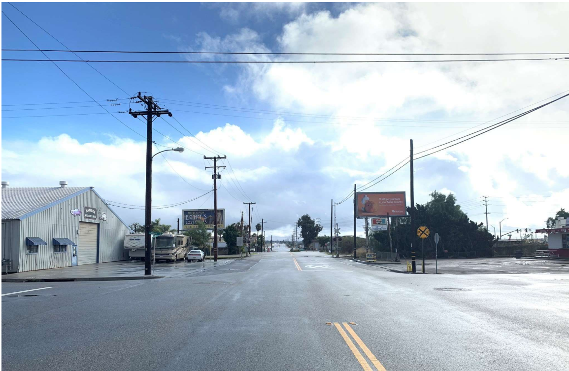
The existing sidewalk facilities are not continuous and some lack crosswalks and curb ramps. Photo taken at intersection of Azahar Street and Los Angeles Avenue
