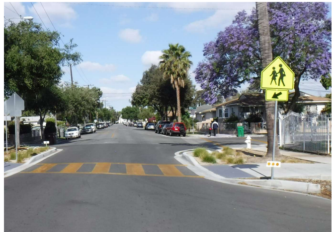
High-visibility Crosswalk, such as the “continental” ladder lines used here. This crossing also features a curb extension to reduce crossing distance and reduce exposure to vehicles and curb ramps for ADA compliance. There is additional notification signage for pedestrians as landscaping.
