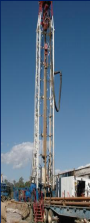
Drilling for local groundwater
