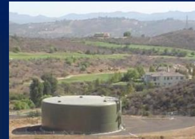
Recycled Water Reservoir WWD No. 1
