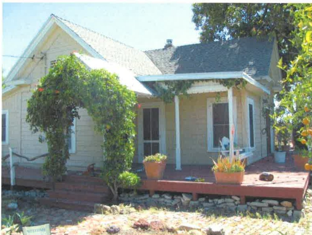
Photo #2 West Elevation (Living room, bdrm#1, and kitchen)
