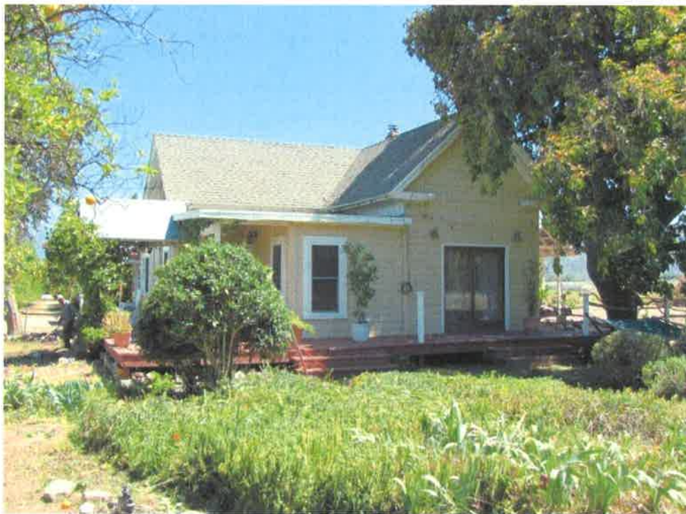
Photo #1 South Elevation (Living room area)
