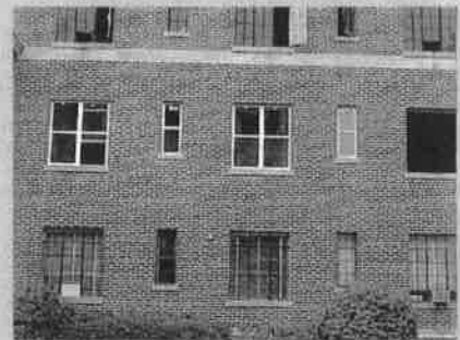
Historic steel casement windows are in the process of being replaced with new units that compromise the character of this building facade.
