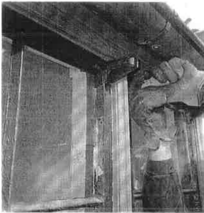
Figure 5. Before realigning the window, paint, caulk, weatherstripping and rust were stripped from all surfaces where the sash and frame were in contact.
