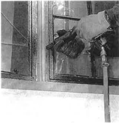
Figure 8. A pneumatic needle gun was used to strip much of the paint from the steel frame and sash. It was followed by wire wheel and small disk sanders and hand chisels. The blunt tipped needles did not damage the steel or adjacent glass.
