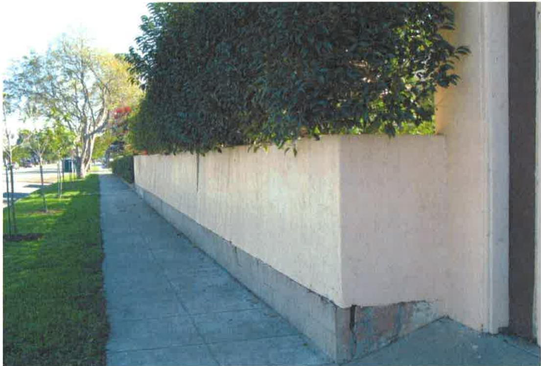
Existing 85 foot long by five foot high plaster wall
