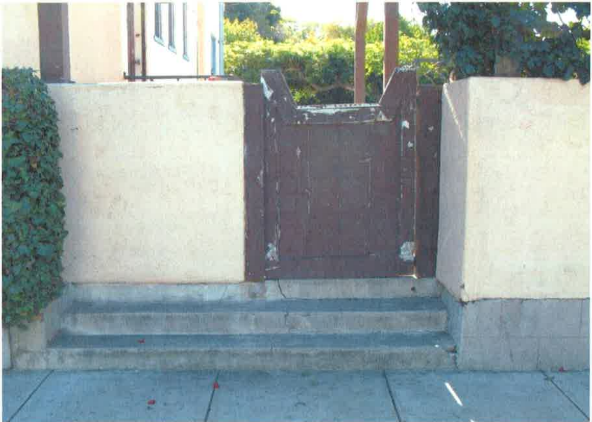
Existing gate and wall.
