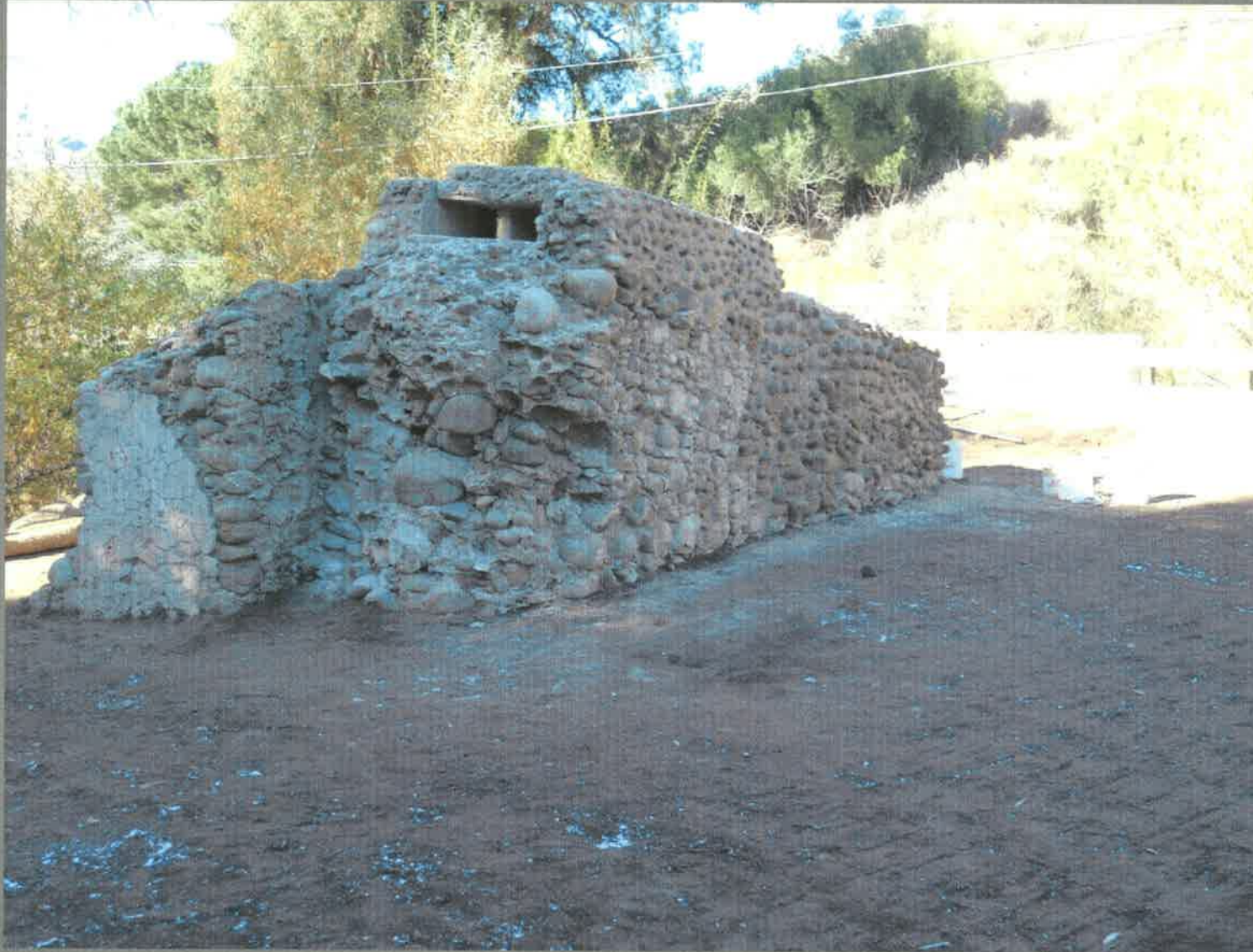
North facing view of restored masonry with grading completed
