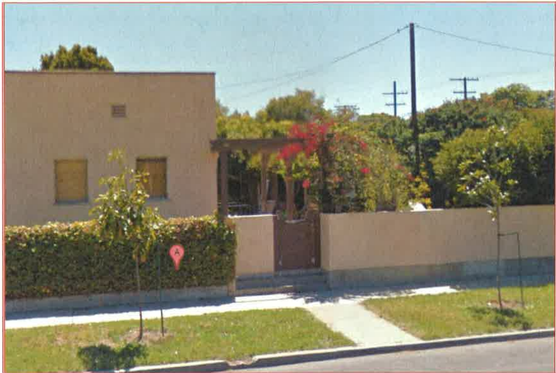
Existing Trellis/Arbor above gate
