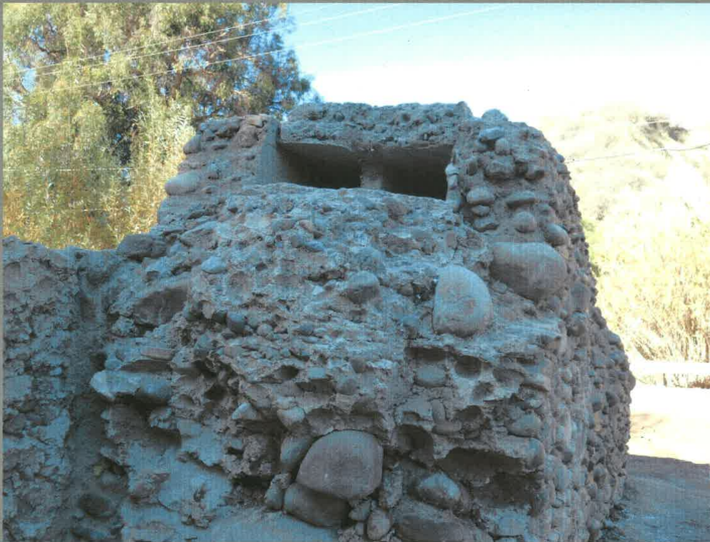
Restored channel of damaged segment looking north
