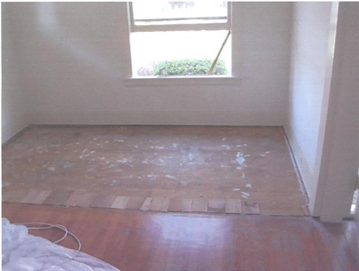
The flooring that was under the carpet was plywood.
