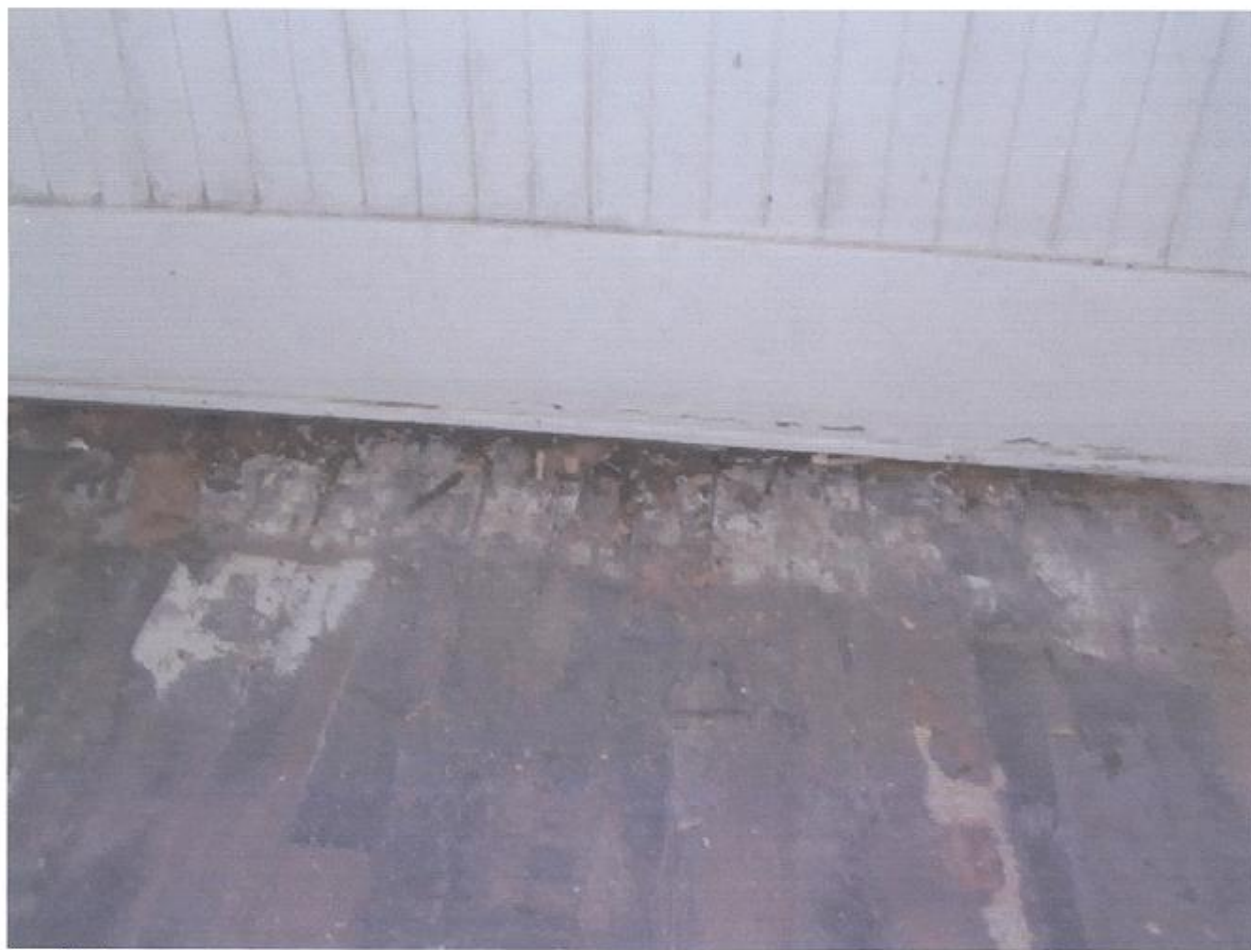
Termite damage
