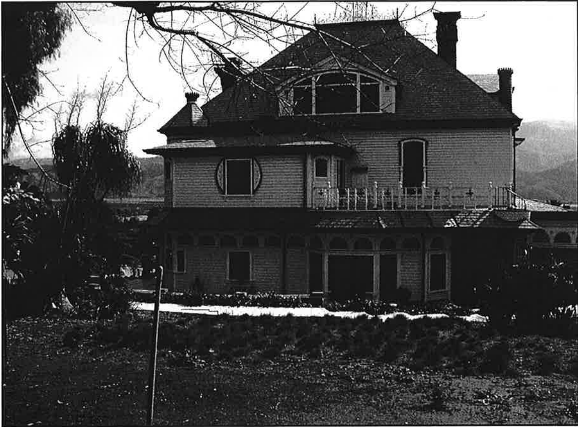
Photo 11. Rear (northern) elevation, Judy Triem, photographer [January 31, 2007]
