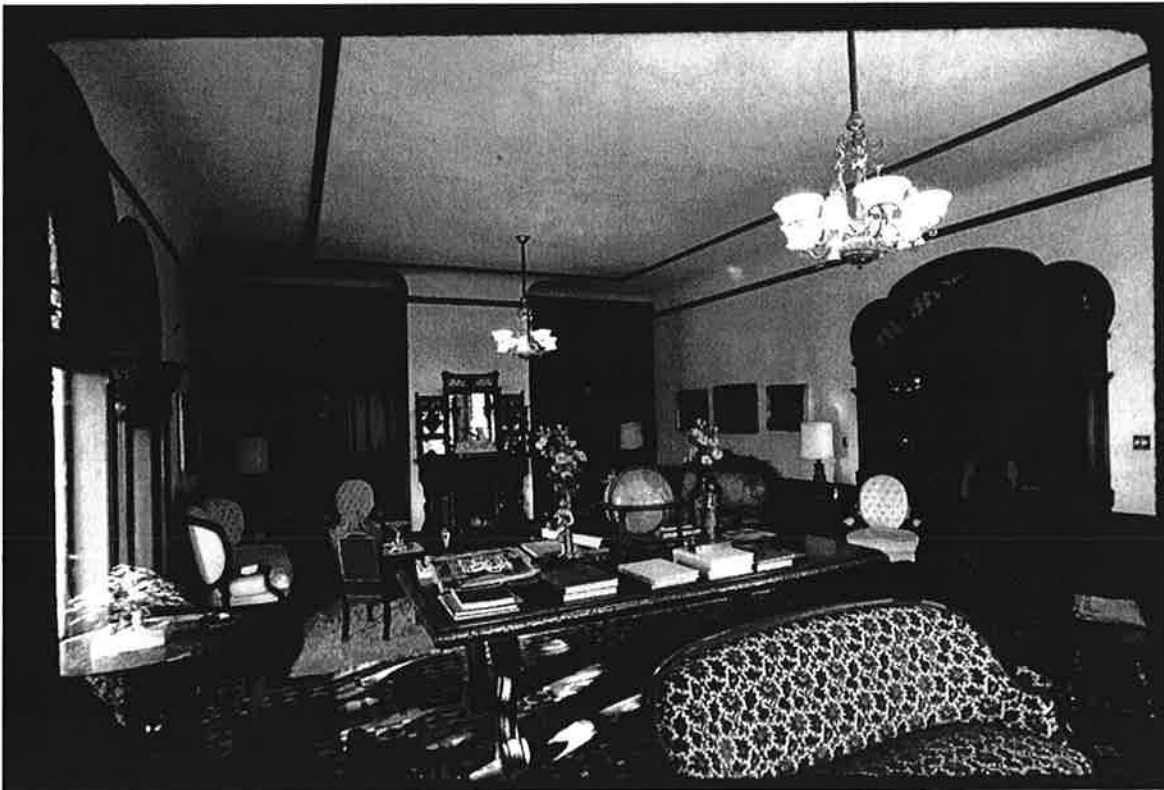
Photo 4. Interior parlor, pre-fire, Phil Hardison, photographer [1980]
