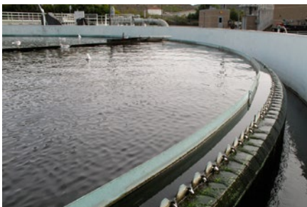
Ojai Valley Sanitary District Wastewater Treatment Plant
