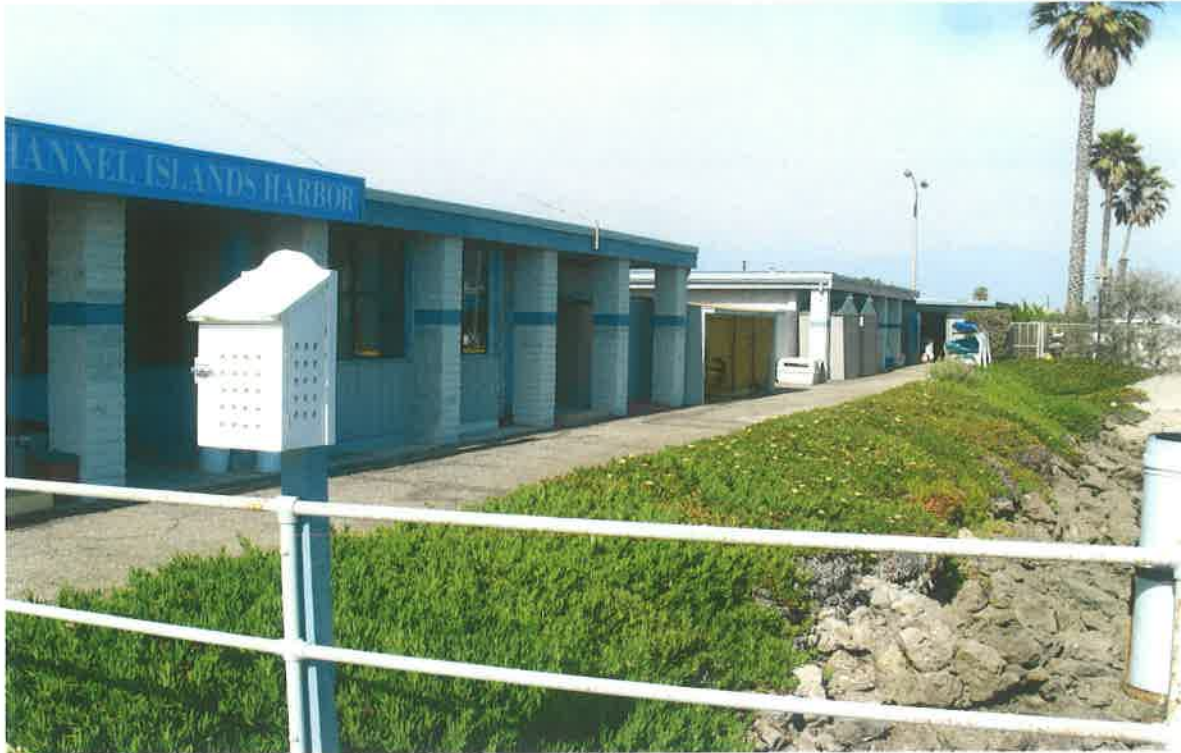
South elevation from gangway.
