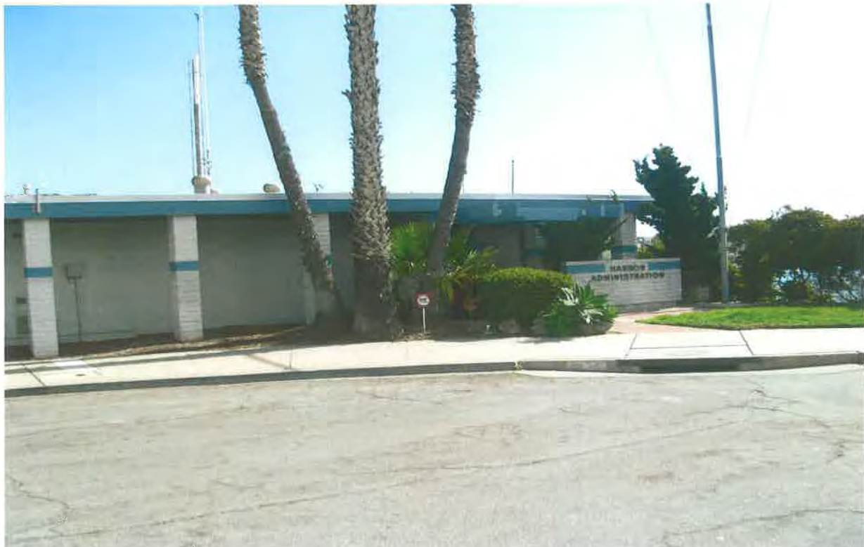
North elevation of Harbor Patrol building from center of Pelican Way. These three Mexican Fan Palms will be retained or replanted onsite.
