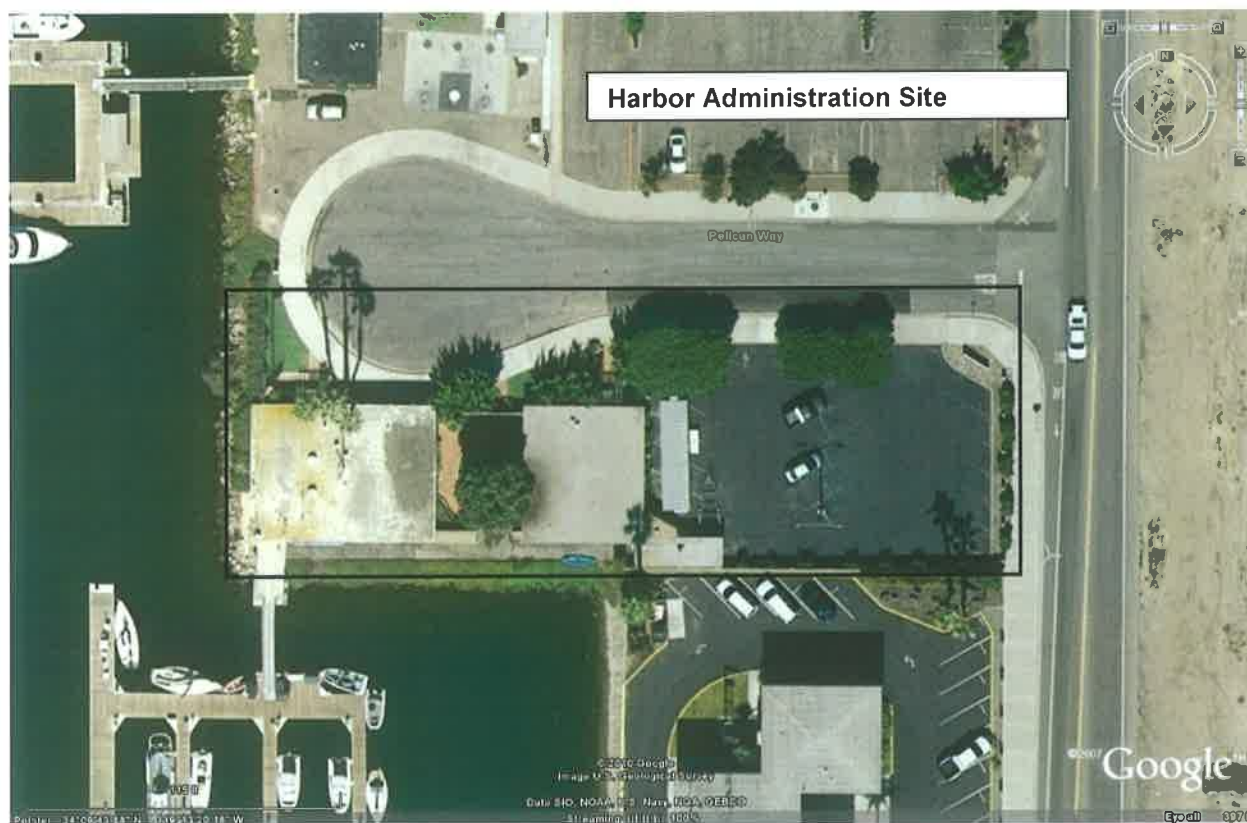
The County of Ventura Harbor Department Administration Building is located on a 21,623 square foot site at the southwest corner of South Victoria Avenue and Pelican
