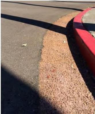
Currently pervious pavement and gutters have been installed at parking lots A and B at the Government Center. Pervious pavement and gutters allow for more water penetration into the water table rather than the water being wasted as runoff. Future pervious pavement and gutter projects have been approved for the entire Government Center complex. GSA is partnering with the Public Works Agency to provide maintenance to the pervious pavement installed in the
