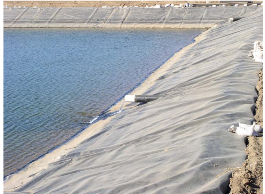
Irrigation tail-water return systems to collect, store, transport and re-use irrigation tail-water
