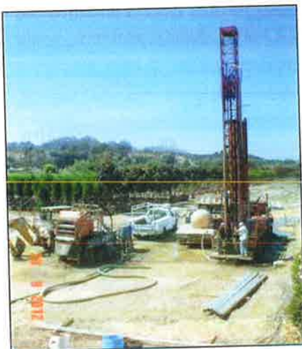
Drilling a test well for the Ventura County Waterworks Moorpark Desalter
