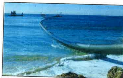
Ocean Outfall Construction
